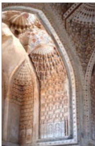
Figure 6 Plaster Cornicing of Timori Era, Roof of Goharshad Begum’s Mausoleum
